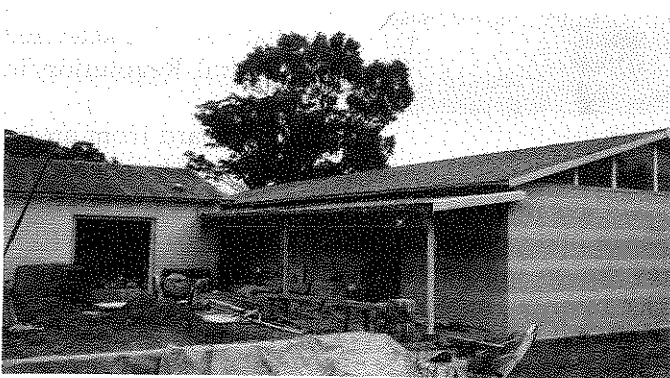
The Soshisha Center for Minamata Disease under construction
