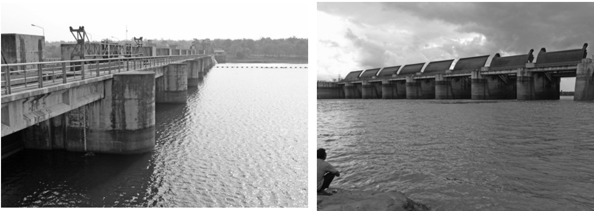
The Pak Mun Dam When the gates are closed (left) and opened (right)
