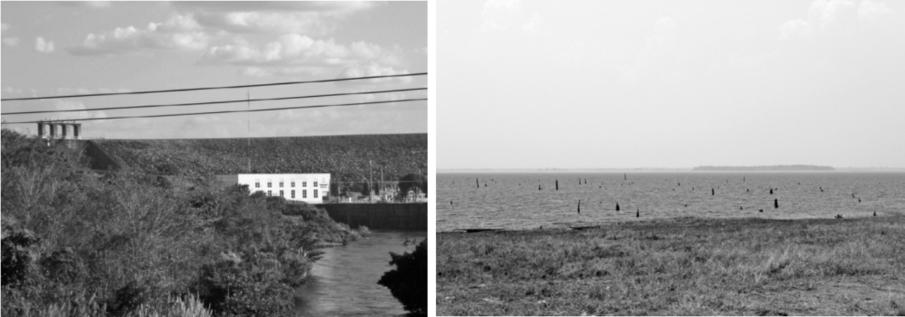
Sirindhorn Dam (left) and its extensive reservoir (right)
