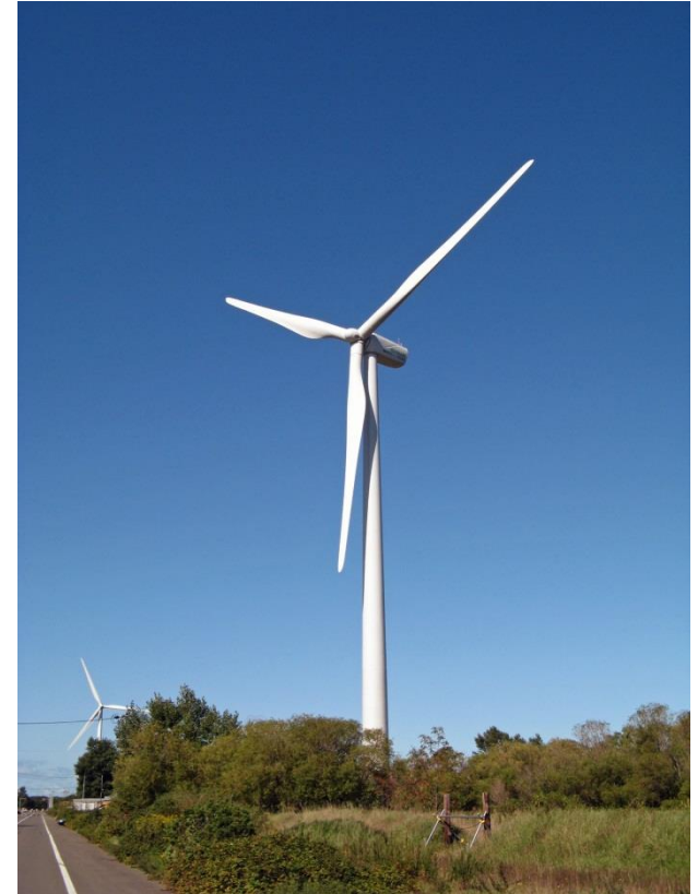
Ishikari Community Wind Power Plant Service commended in January 2008
